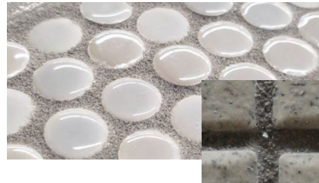
UnsanDED Grout: No visible aggregate and a smooth joint
