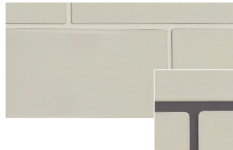
UnsanDED Grout: No visible aggregate and a smooth joint
