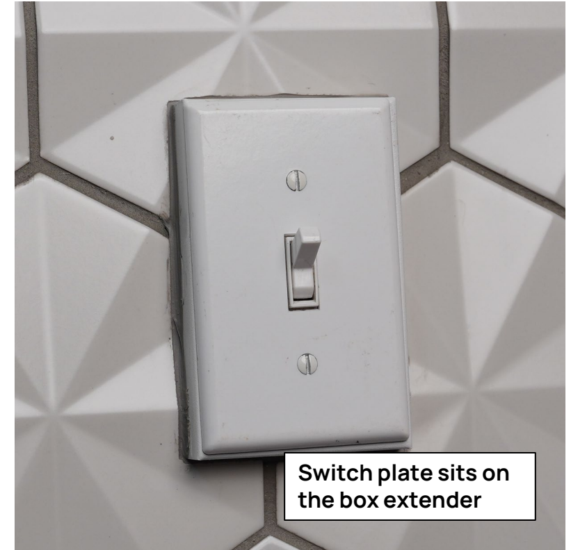
3D Tile with electrical box: tile is cut tight
